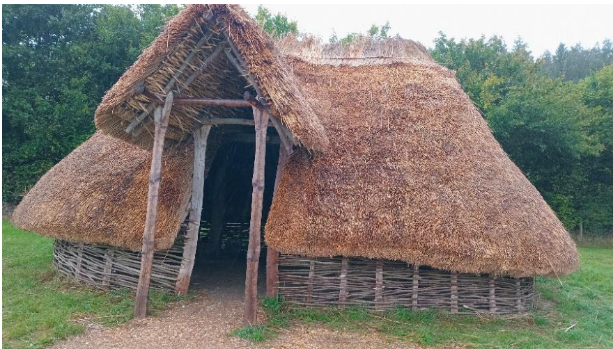
Neolithic – the reed thatch is very thick but smoke from the fire can filter out through it.
